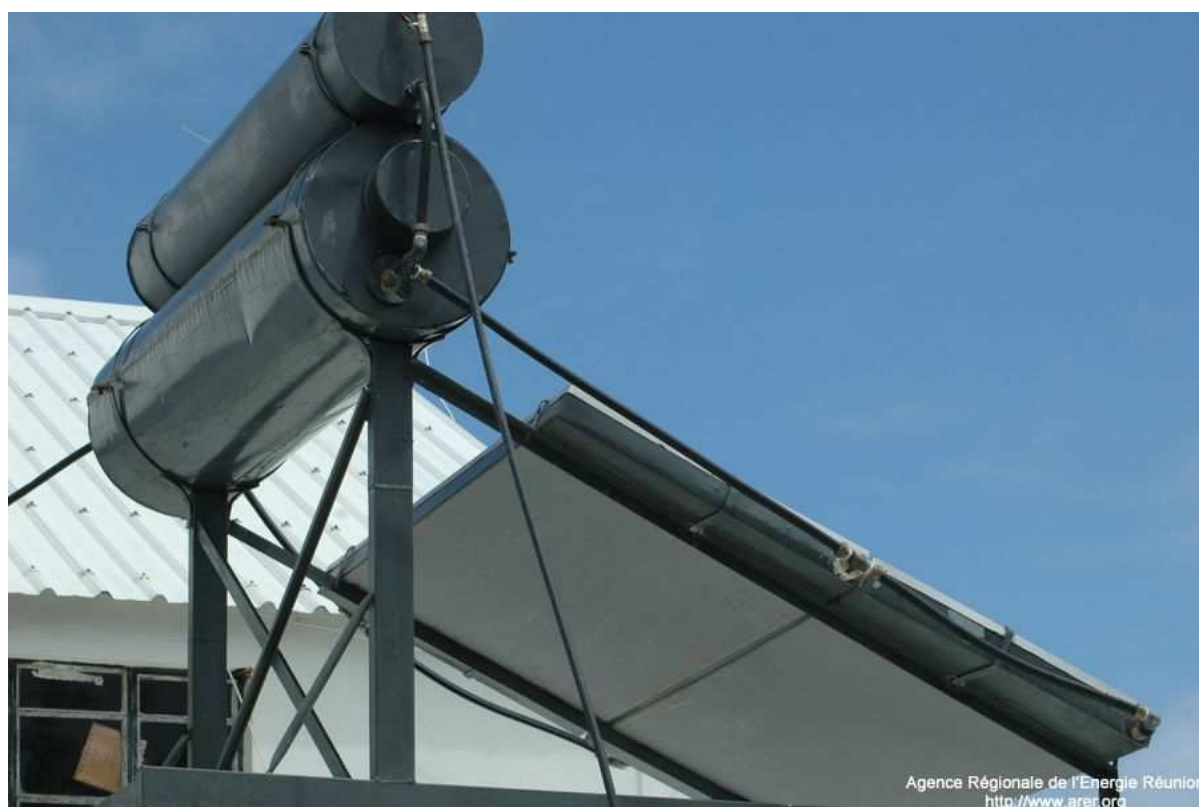
Figure 22: example of actual type of solar water heater installed on Rodrigues Island
